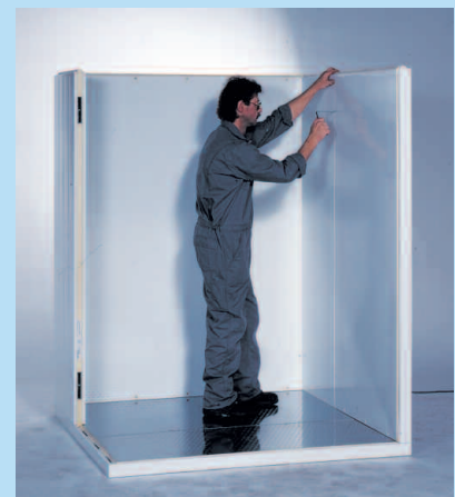
Simple assembly of the panels
